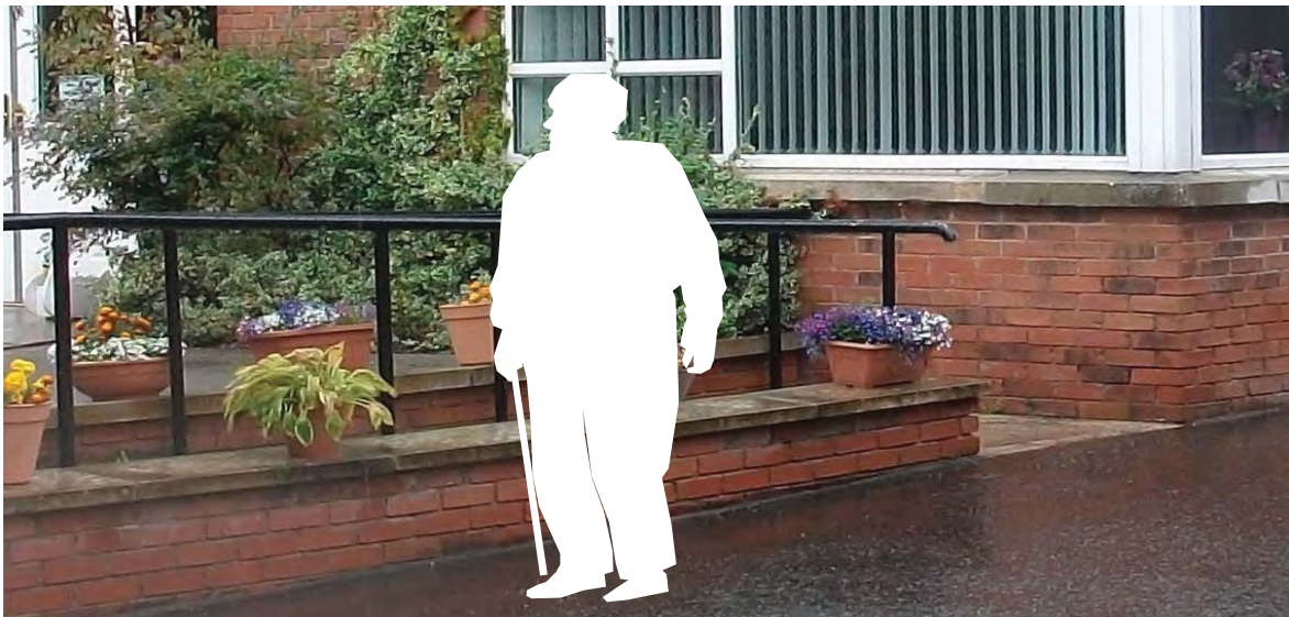
12 Steel handrails to exterior ramp.
