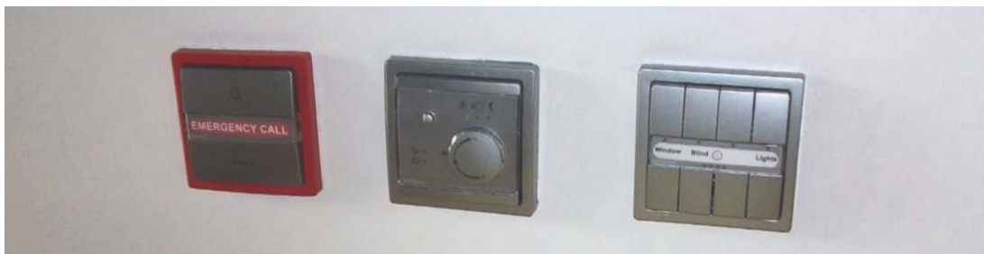
10 Heating controls along with alarm and light switches beside
