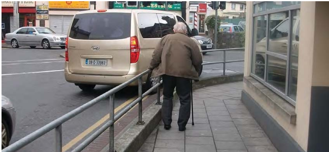
13 Metal guarding between carriageway and footpath.
