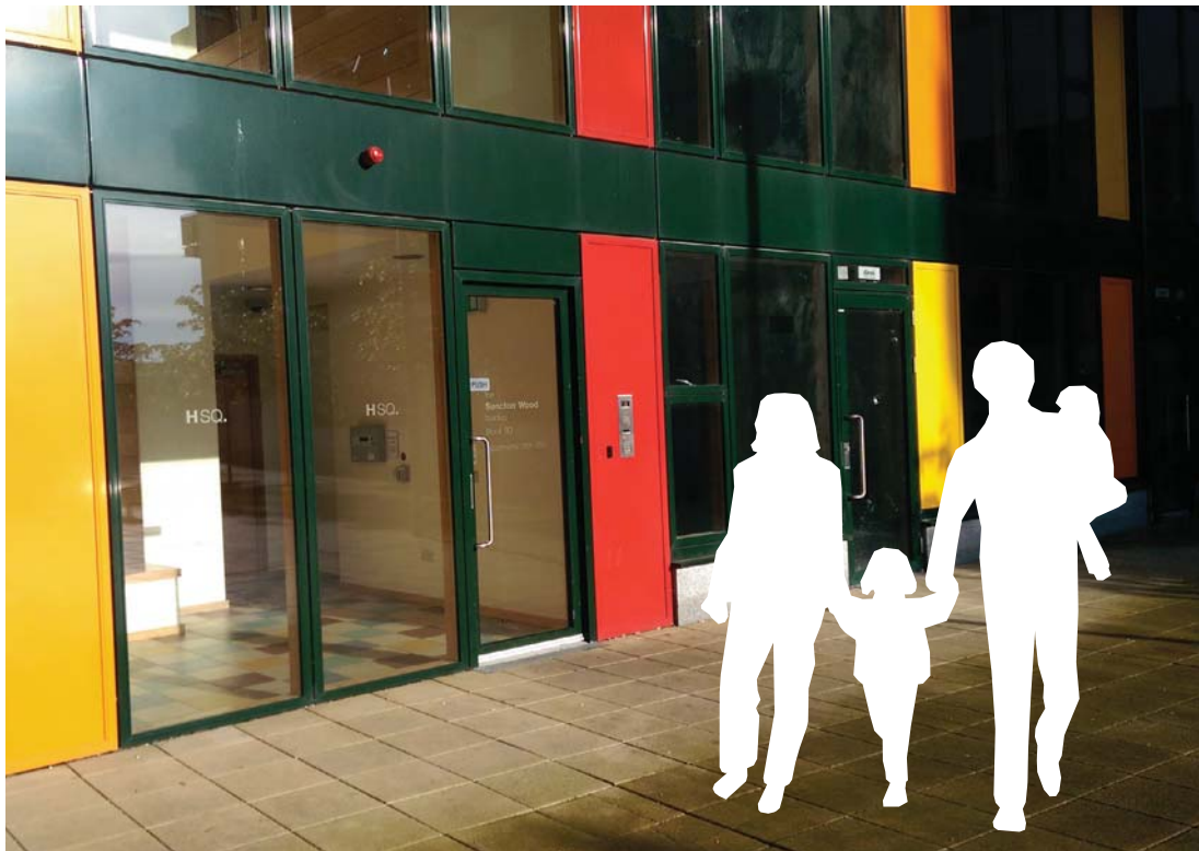
05 Entrance to a contemporary apartment block.
