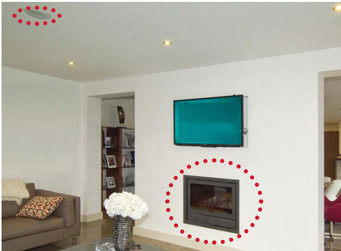
22 Living area with a sealed stove and an air supply vent on the ceiling.
