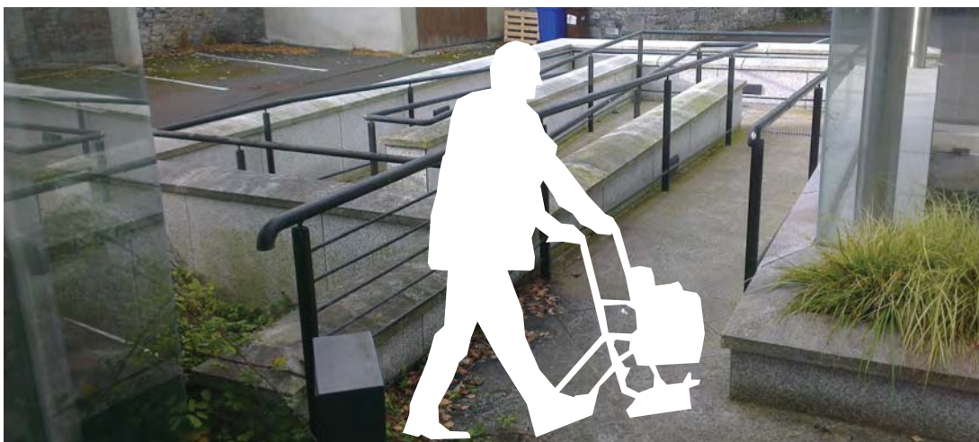
11 Complicated ramp at the main entrance to a building that may be confusing.
