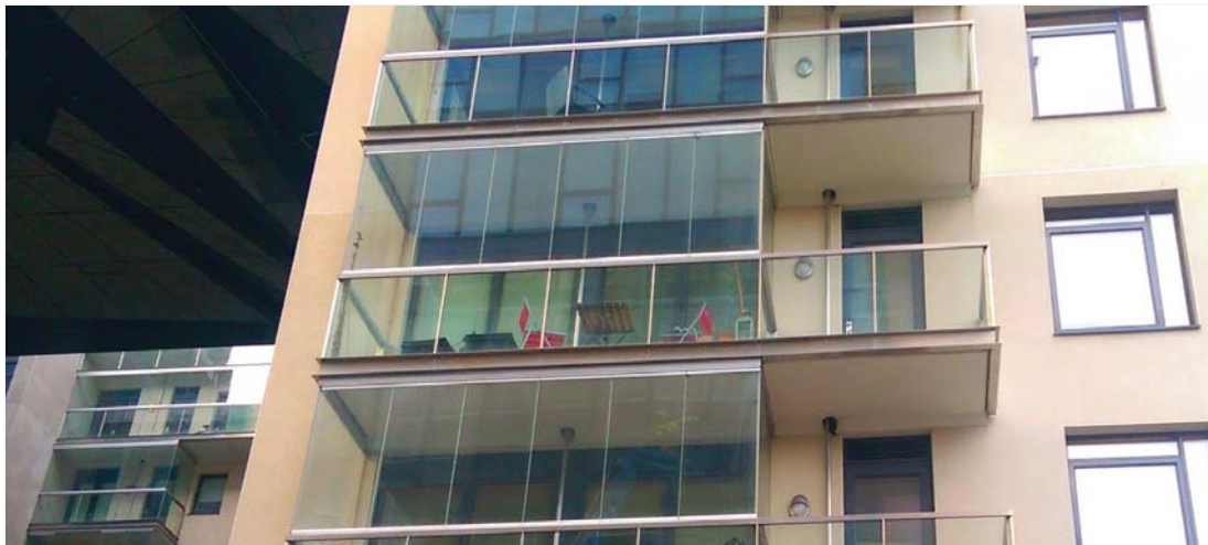
14 Fully glazed balcony or 'Winter garden' in a recent apartment development. This also has a smaller open section with direct access from a bedroom.
