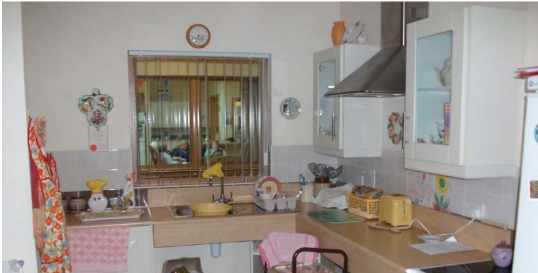
05 Clear glazed wall-mounted kitchen units giving visual access to contents.
