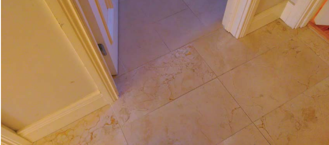
04 Door threshold between tiled hallway and tiled bathroom.
