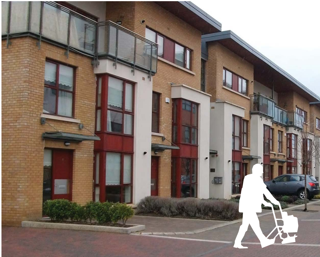
01 Entrance doors to three storey townhouses.
