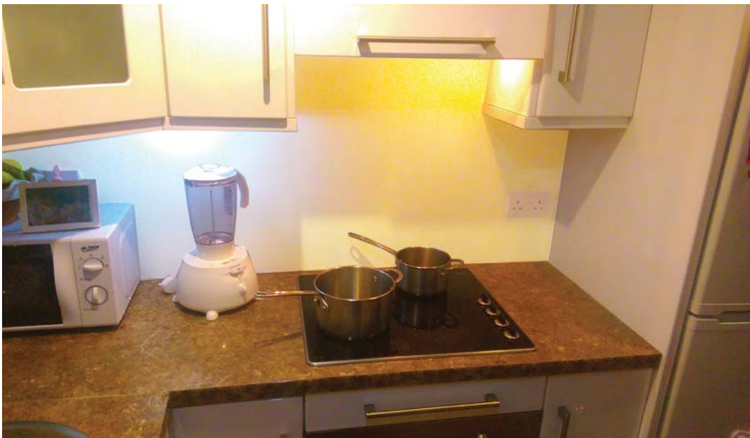
20 Lighting fixtures fitted to underside of wall mounted kitchen units.
