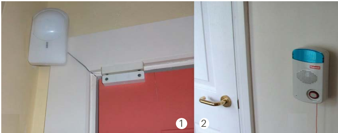
33 Image 1 to the left, shows an exit sensor that sends a message to a control point (family member, carer or care provider) when the door is opened. Image 2 on the right, shows an emergency call unit with a push button and a pull cord.
