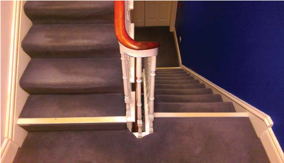
12 Internal domestic stairs.
