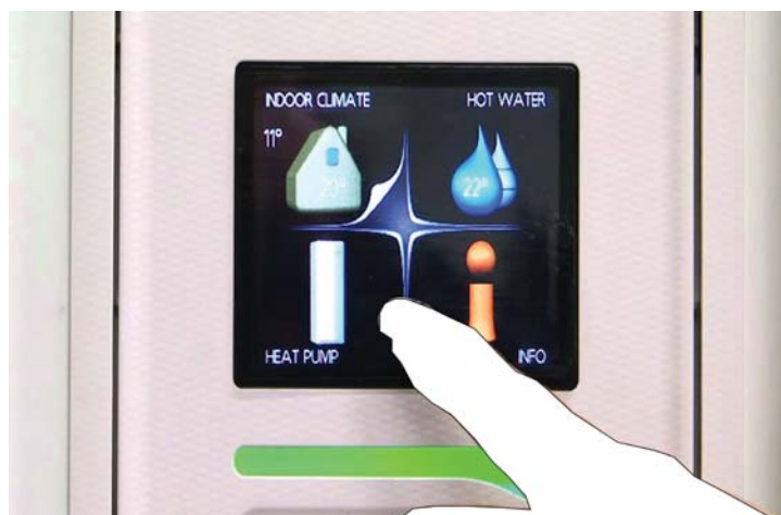
24 Example of an advanced space heating, water heating and ventilation control panel.
