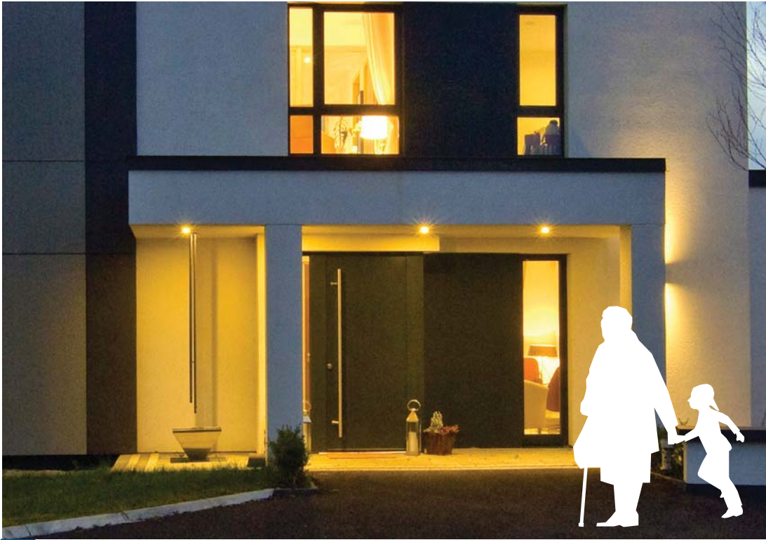
02 A entrance to a contemporary detached dwelling.
