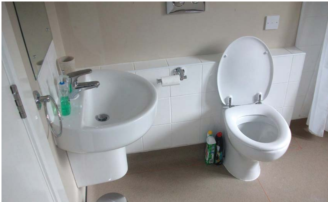
07 Contemporary bathroom fittings in an accessible bathroom.
